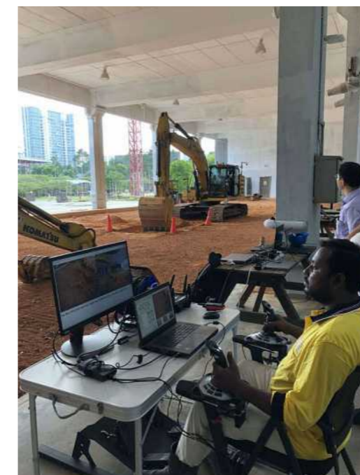
Teleoperation of excavator trialled at BCA Braddell Campus' Excavator Yard.
